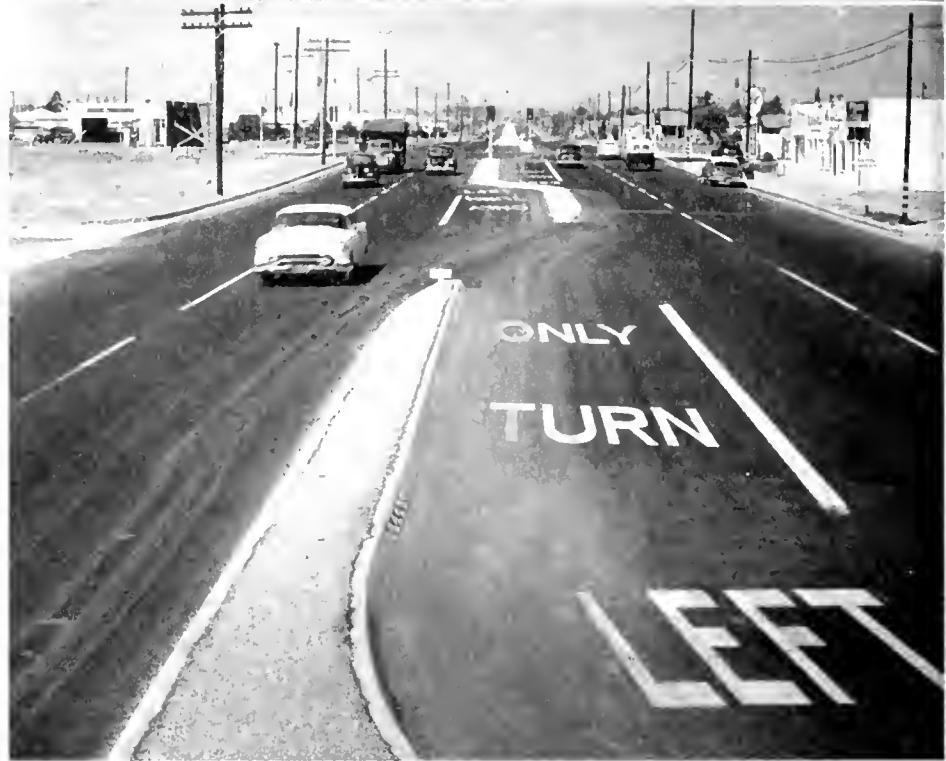
UPPER: Looking westerly along State Highway Route 175 from Inglewood Avenue showing East Redondo Beach grade separation with Santa Fe Railroad. LOWER: Looking westerly along State Highway Route 175 showing intersection with Crenshaw Boulevard. This photograph shows construction details in central dividing strip in order to provide for left turning traffic movements.
